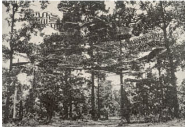
FIGURE 9. Where short stretches of concealed roads have sparse overhead cover, they may be concealed completely by overhead screens tied between trees and garnished to match the surrounding foliage.
